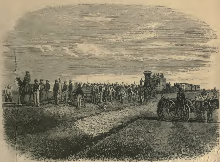
Laying the Track.
